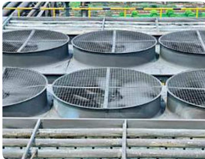
Cooling tower fans are applied throughout the downstream industry and pose specific maintenance challenges for which SKF has developed a broad range of solutions.
