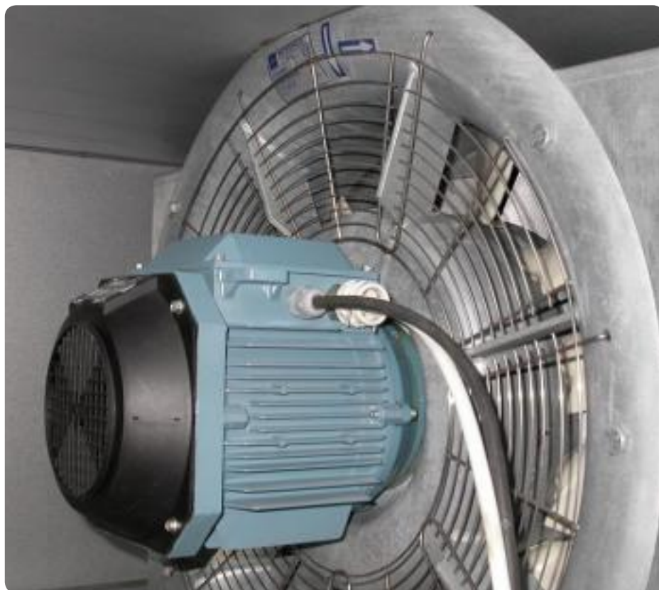
Fan installation at Sunderby hospital
