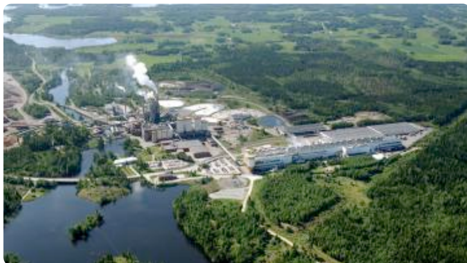
Aerial view of AssiDomän Cartonboard AB in Frövi, Sweden
