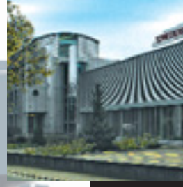
Roggwil, Switzerland Main company domicile and production facility
