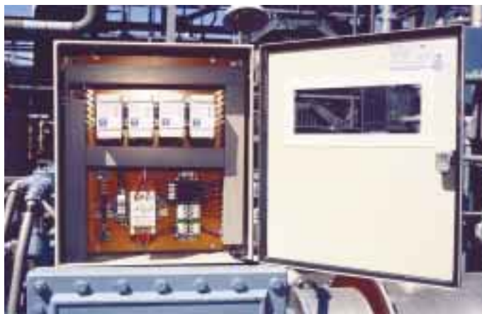
Electronic cabinet with built-in MCM™ units
